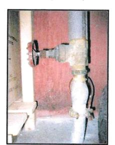
Exhibit 5-2: Example of Wiped Lead Joint
